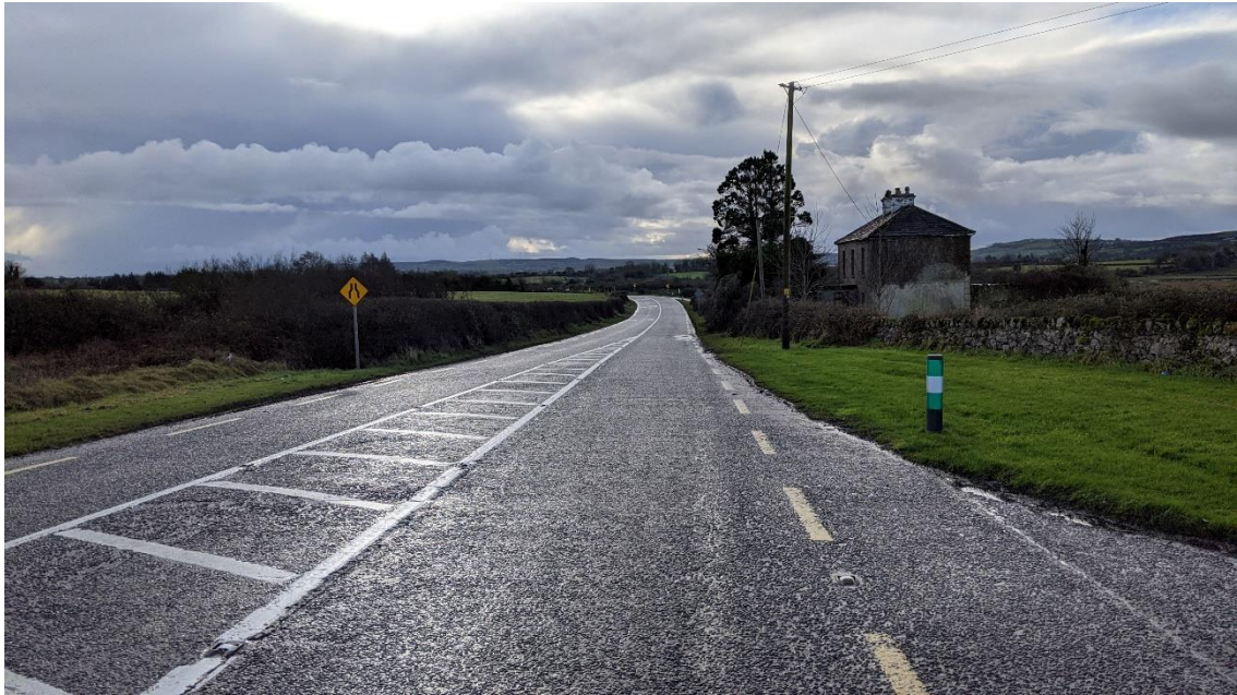
Figure 14.3: N69 at Glenbane East
