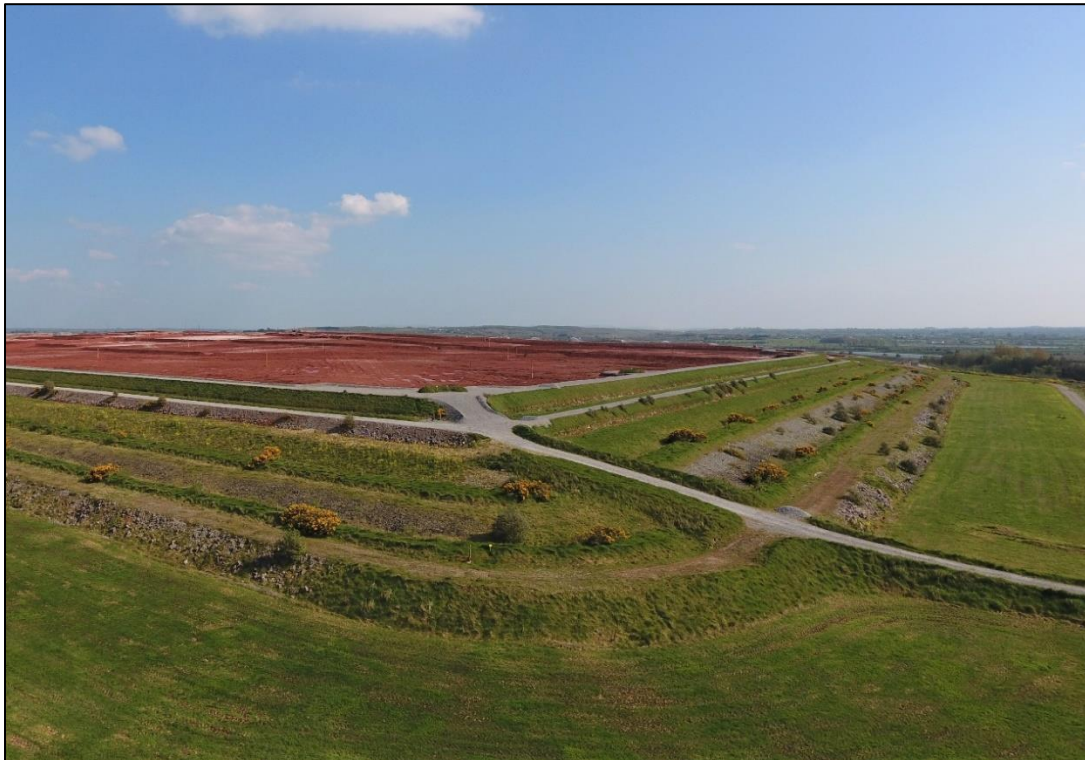
Figure 8.16: North and West Sectors of the Phase 1 BRDA (April 2021)
