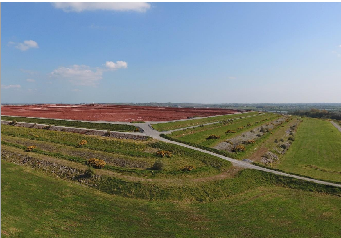
Figure 10.51: North and West Flanks of the Phase 1 BRDA (April 2021)
